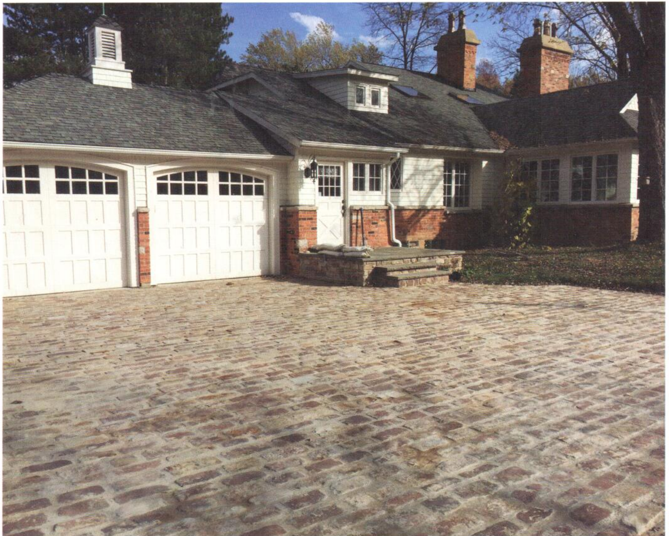
Experienced Brick & Stone supplied the materials for this Medina sandstone driveway (above) and this bench made from sandstone curbing (below), both found at homes in Williamsville.
